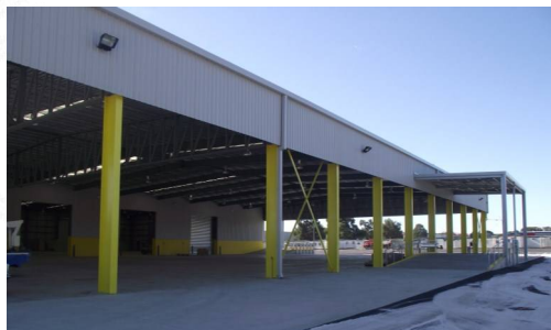
Company Brand Coloured Steelwork
